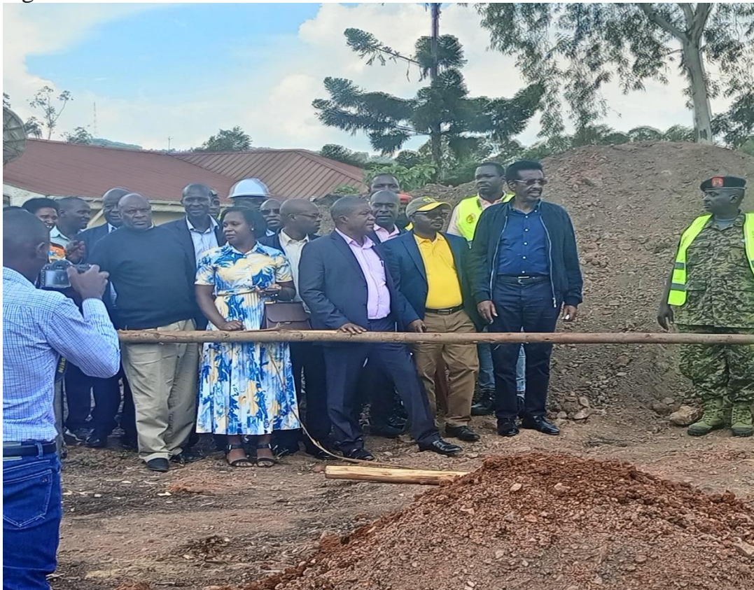
Chief guest, Area MP, RDC and other guests inspecting the theatre site
